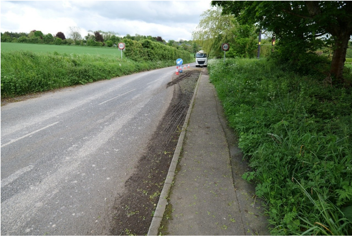
A3. May 2025 - Tanker stationed at Aldworth Road Pumping Station
