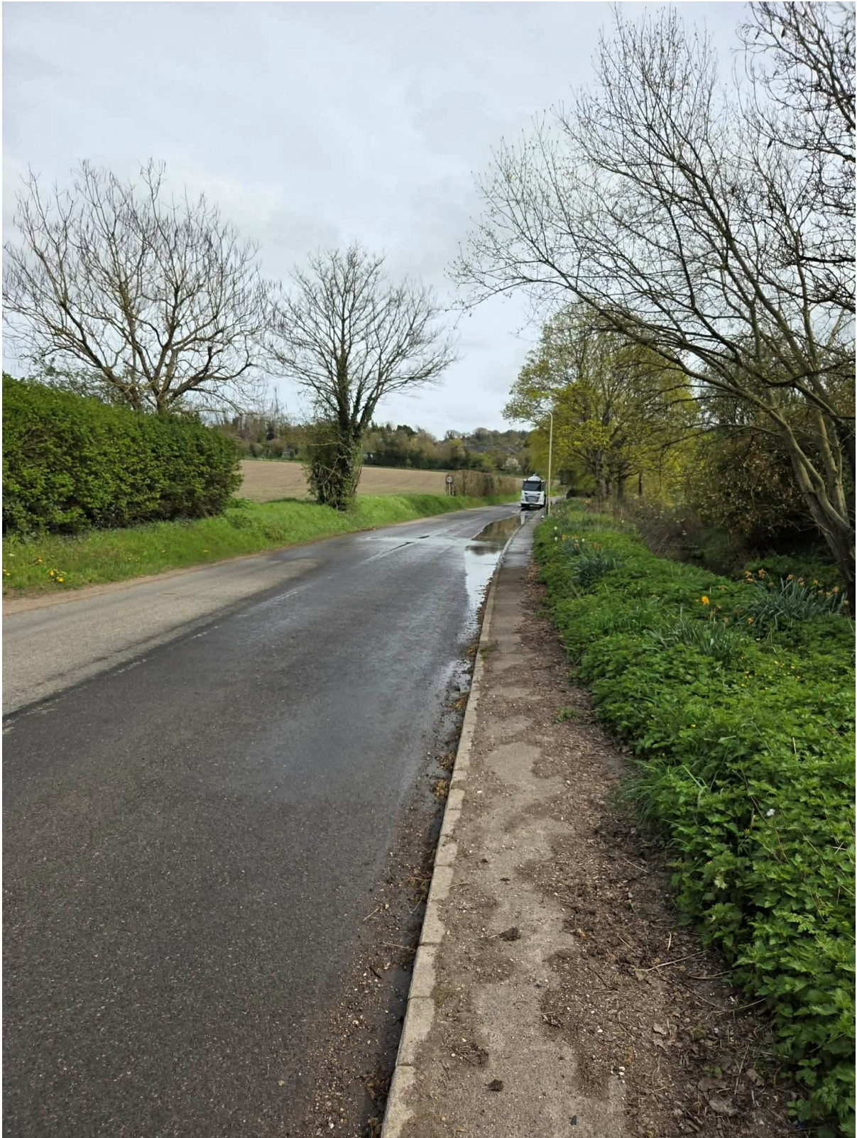
Figure 1: Tanker operating at Aldworth Road pumping station, 4 th April 2026
