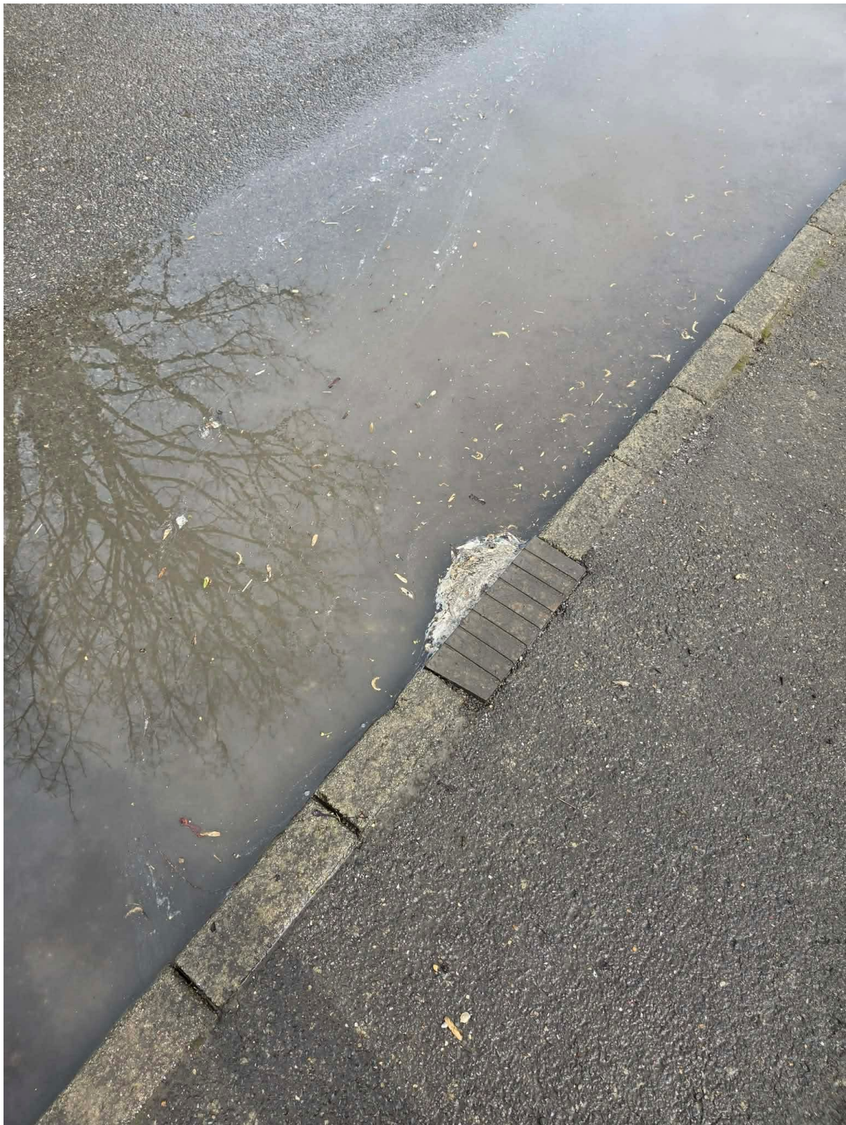
Figure 3: Evidence of surcharge residue on Aldworth Road adjacent to the pumping station, 4 th April 2026.
